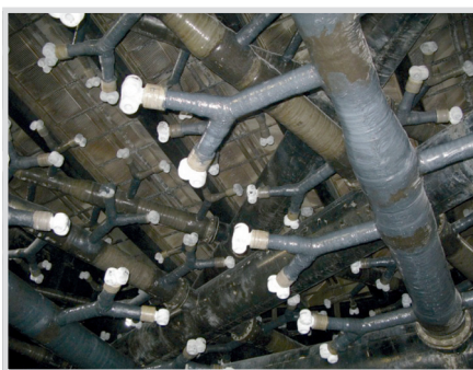
Fig. 5. Orientation of nozzles
