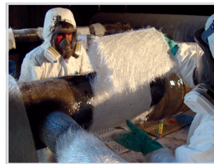
Fig. 6. Lamination of Y-Connectors.
